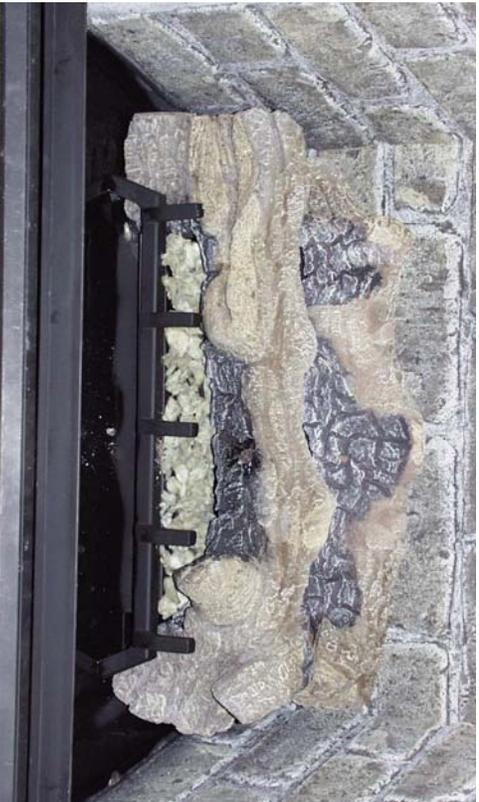
**Step (6)** Place rear log on to the log retainer 1/2" away from back of fireplace. (If refractory liner is used, make sure refractory liner is installed first then back log is to be pushed up against it as tight as
