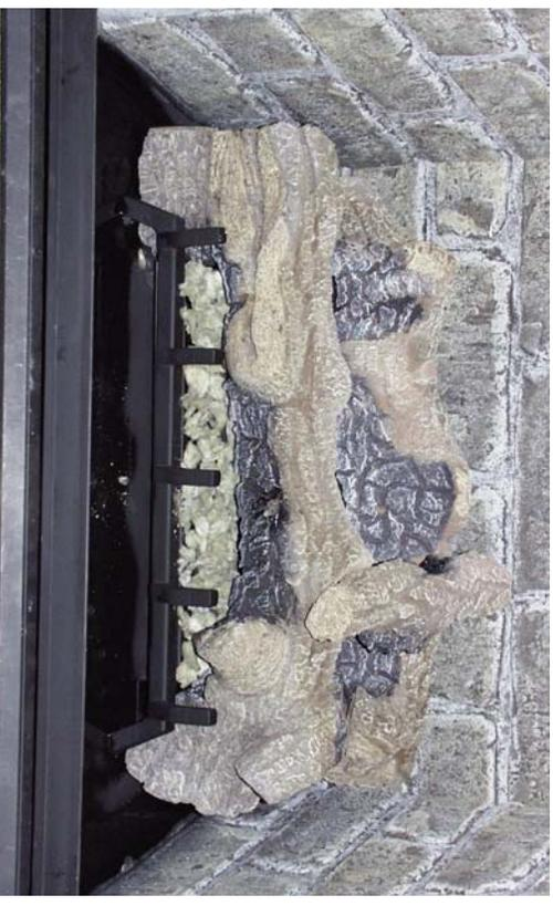
**Step (7)** Place right crossover log across front and back logs using the log placement pin as a guide.
