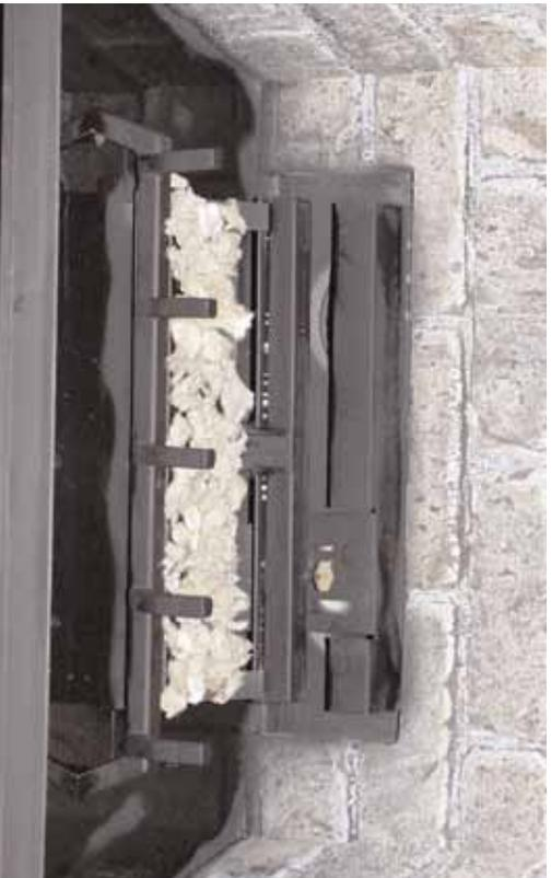
**Step (4)** Break glowing embers into thumbnail size. Place glowing embers on to the surface of the front burner, to the surface of the ember plates and over crossover to the same height as ember plates. Height on front burner 1/2" to 3/4". Height on ember plates 3/4" to 1". Do not cover back air openings on ember plates.
