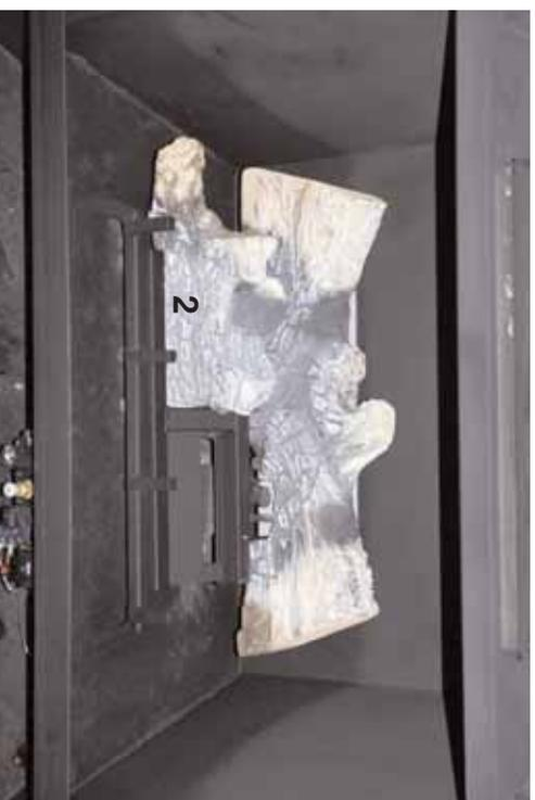
**Step (2)** Locate flat surface on Log (2) and place directly onto left ember plate, push log fully to the right until it touches the crossing-tube.
